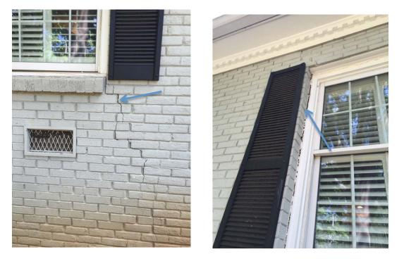
The photo below shows the window at the left rear bedroom at the rear wall where patched mortar was observed.
