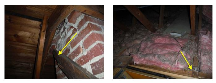
The roof trusses are site built, and although intended on spanning from the front exterior wall to the rear exterior wall, they are likely relying on the interior walls for bearing. The lack of a bearing wall between the living room and the dining room is likely the reason for the cracking in the ceiling.
