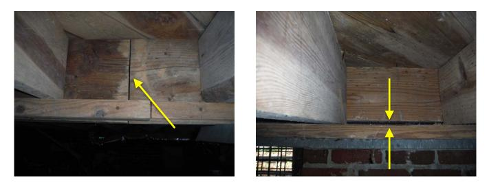
At this time, I recommend a series of repairs including replacing the rotted bands and joists, as well as adding dropped girders under the existing over-spanned joists that are being overloaded by the hall walls. See the attached Foundation Repair Plan "A" for locations and clarification of all recommended repairs.
