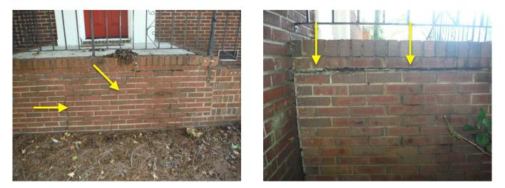
Given the condition of the steps, the cost of repair, the concerns with flashing and the potential for ongoing water damage, I recommend removing the masonry stoop and installing a new front porch. Install the new porch over new concrete footings over solid 2000 psf soil, with new flashing between the porch and the existing band to protect the house band from water penetration, as required by the 2012 NC Residential Code.
